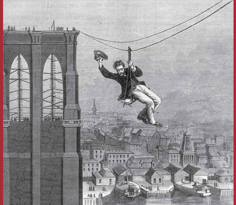
Illustration showing E. Frank Farrington, master mechanic of the construction of the Brooklyn Bridge, sitting in a boatswain's chair secured to a traveller rope, August 25, 1876. ©Stefano Bianchetti/Corbis
